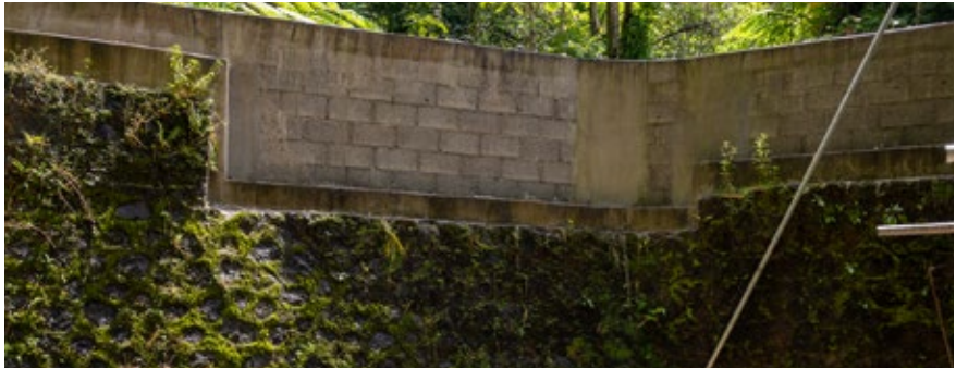
PADU - Extension of River Protection Wall
