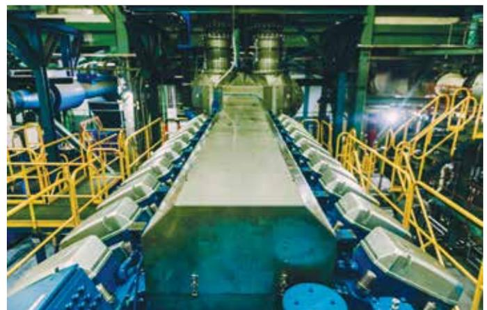
After an 11-week installation period, a new Wartsila 9.7 MW 20V32 engine was successfully commissioned and put into full service in September, increasing the Company's overall power generation capacity to 52 MW. During the installation period, significant civil, mechanical and electrical works were completed.
