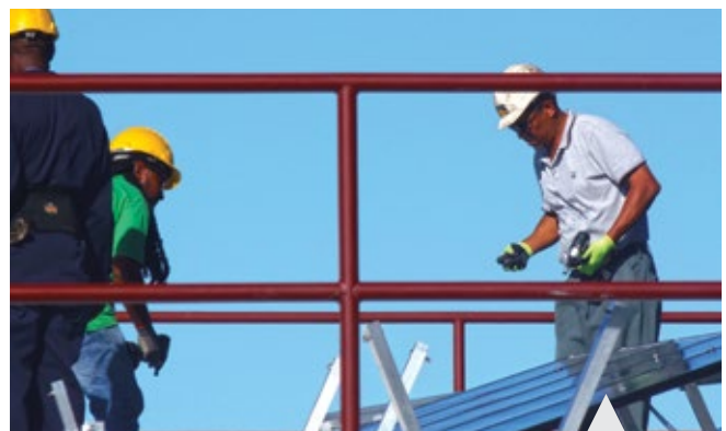
Installation of Solar Panels
