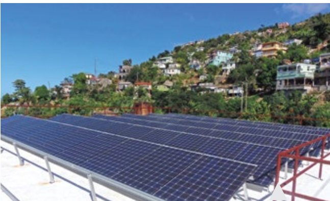
Solar Panels on MAN Units at Fond Cole
