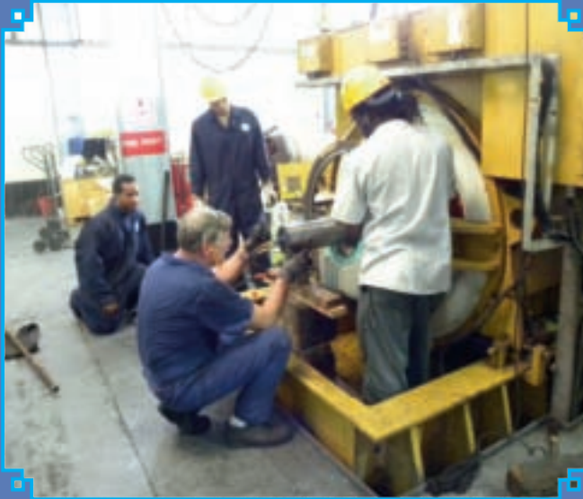
Refurbishment of FC 5
