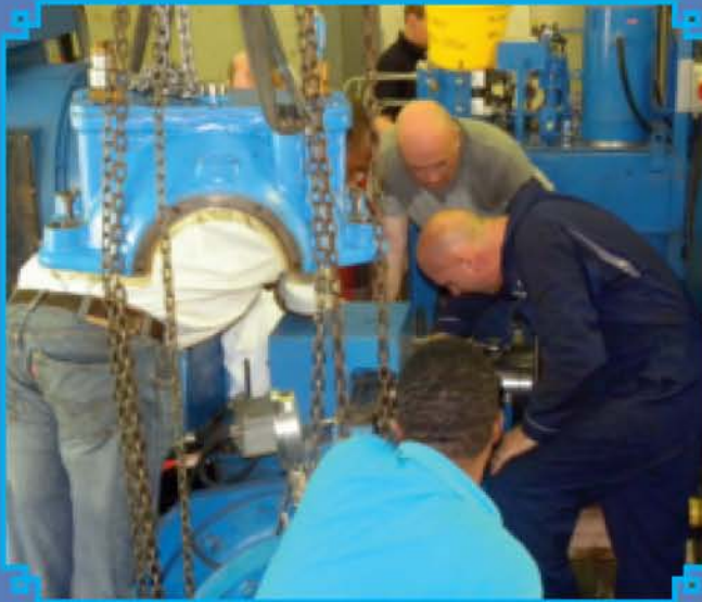
Work on Refurbishment of Padu
