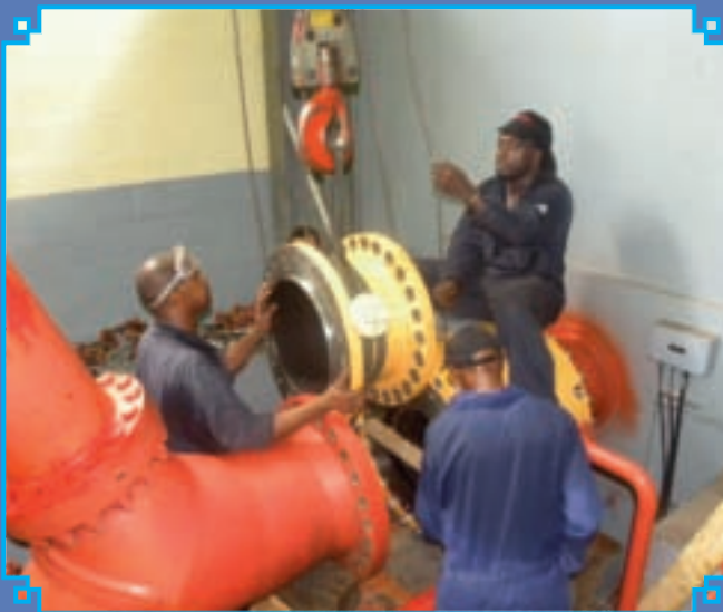
Installation of Spherical Valves at Trafalgar Hydro
