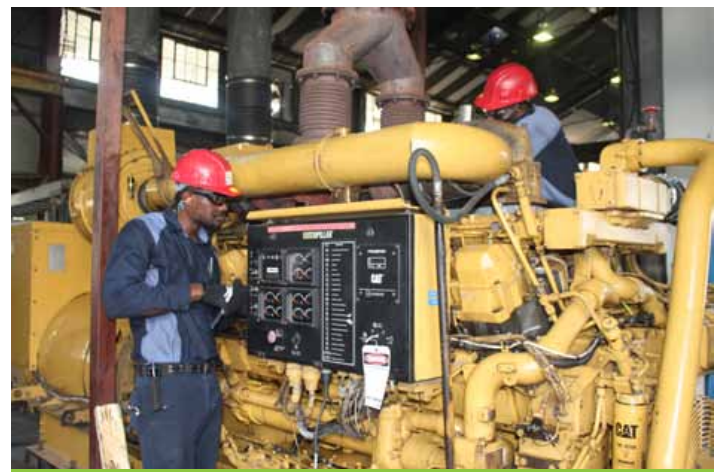
Apprentices fully engaged in overhaul of engine
