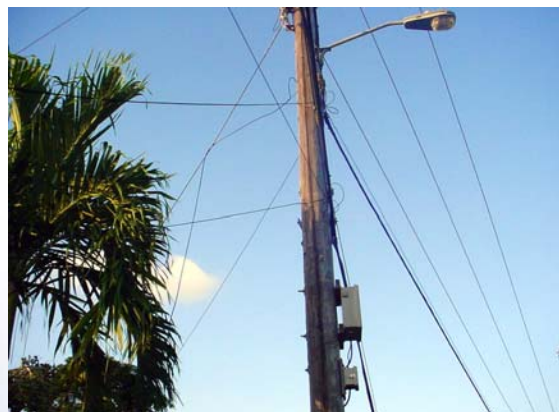
A Remote Terminal Unit; a component of the SCADA system located at Conference, St. Andrew's
