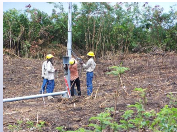
A GRENLEC crew after the erection of the unit
