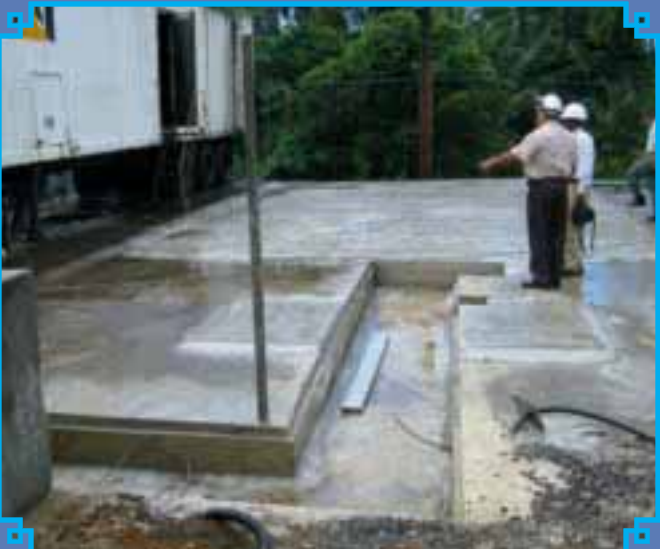
Work to Install the 1.4MW unit at SugarLoaf
