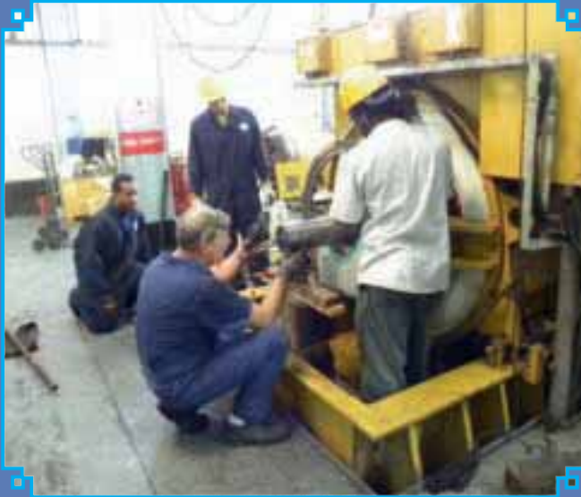
Refurbishment of FC 5
