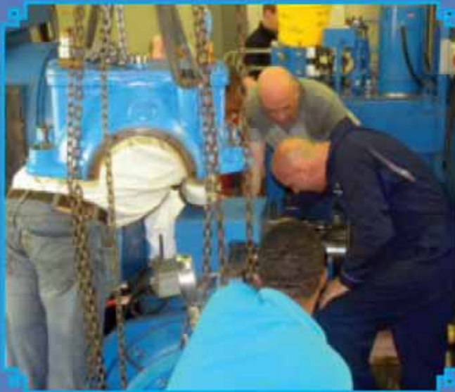
Work on Refurbishment of Padu
