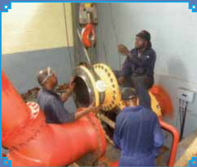
Installation of Spherical Valves at Trafalgar Hydro
