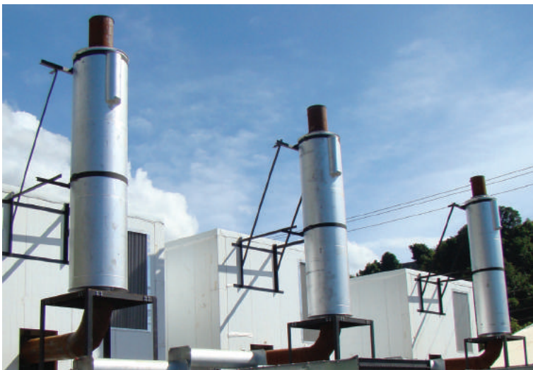
New medium speed generating sets at Fond Cole.
